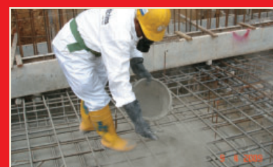
3. Sprinkling prior to casting
